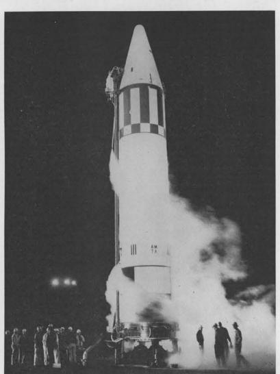
THIRTY MINUTES before firing time of a Jupiter missile vapors surround the "bird." Cables leading off to the left of the rocket carry wires to control Sandia-installed telemetering equipment.
